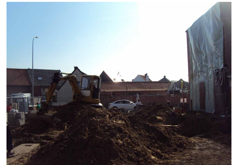
demolition phase block D
